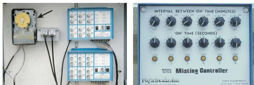
Figure 10-41 Static control systems rely on clocks and timers to manage intermittent mist and fog systems. (a) A 24-hour clock (arrow) turns the system on in the morning and off around dusk, or can be adjusted manually. (b) Time clock controlling the minutes between mist interval "on" time and the seconds of actual mist duration is wired to the 24-hour clock.
